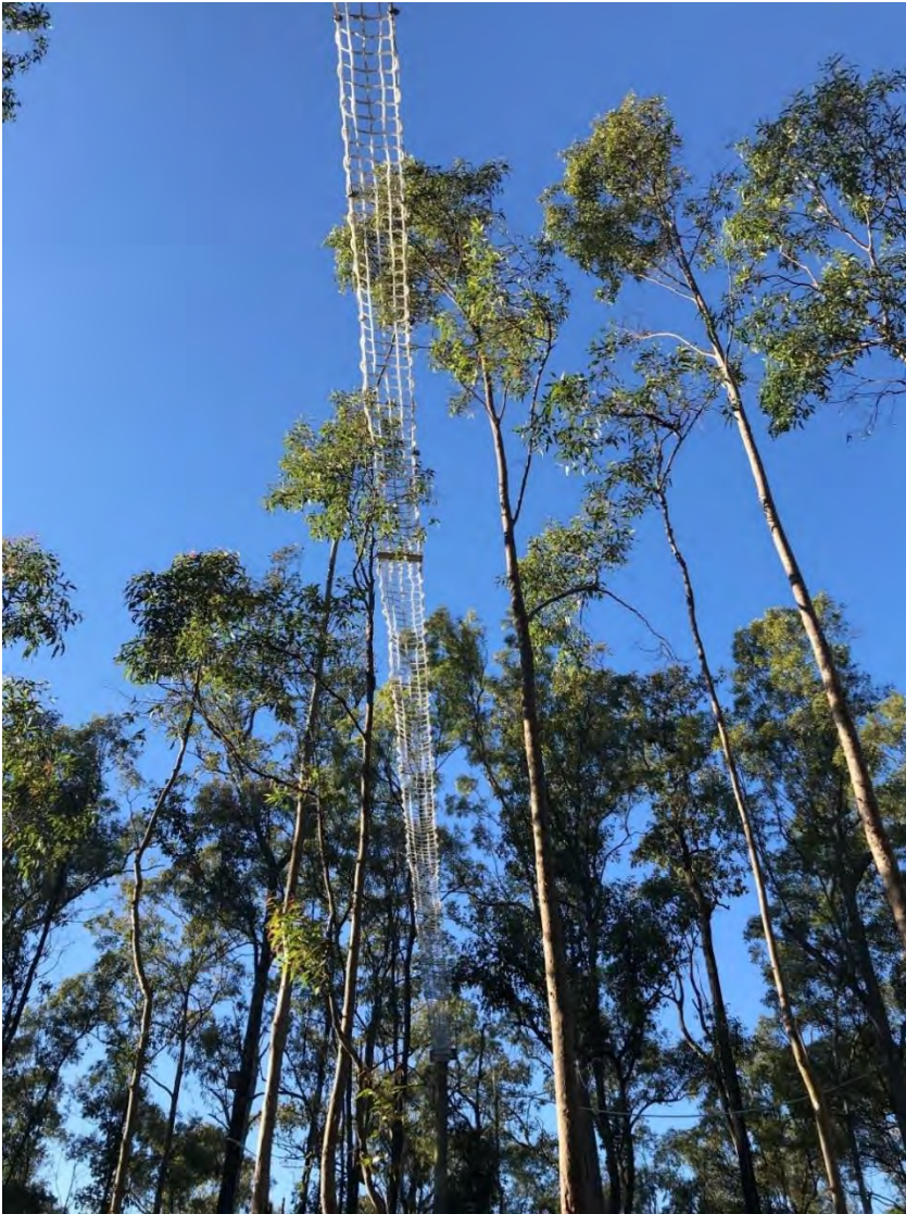
Plate 5.7 Flat rope ladder crossing design Jinker Track, Morton Bay Regional Council (EMM, 2020)
