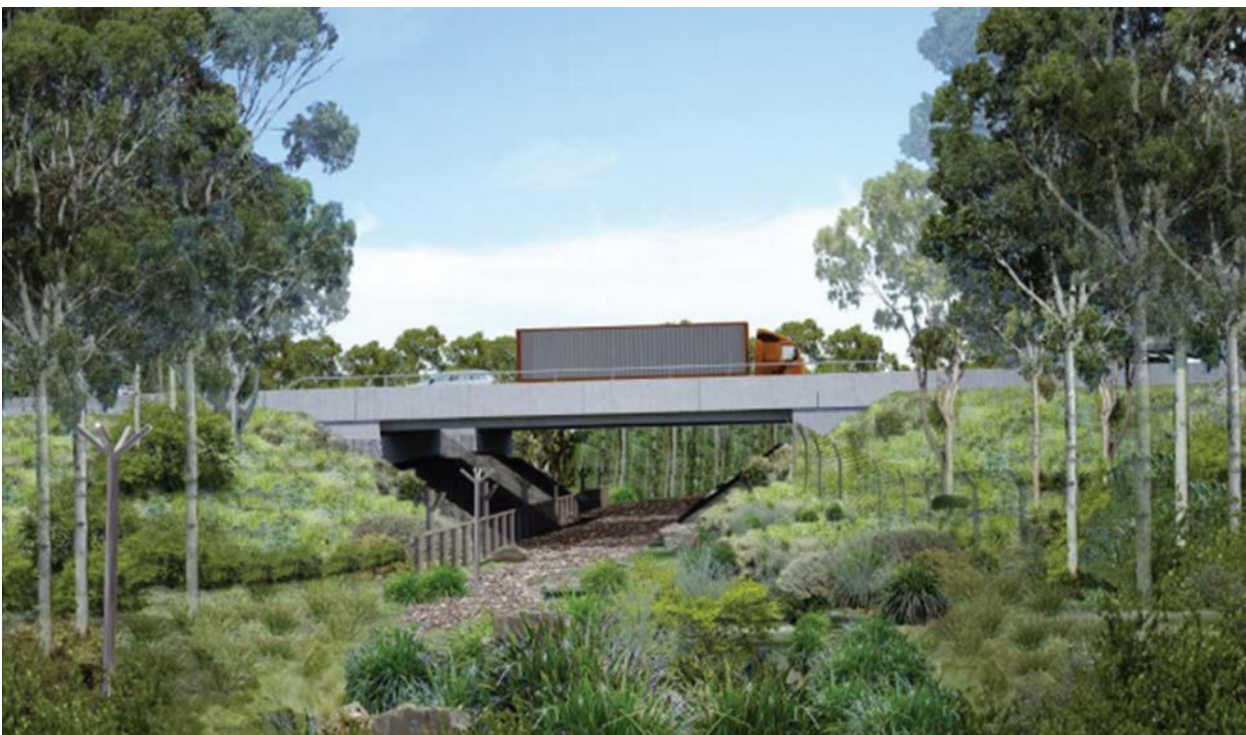
Plate 5.4 Image shows fauna furniture under bridge and fauna exclusion fencing leading up to bridge (RMS 2017)
