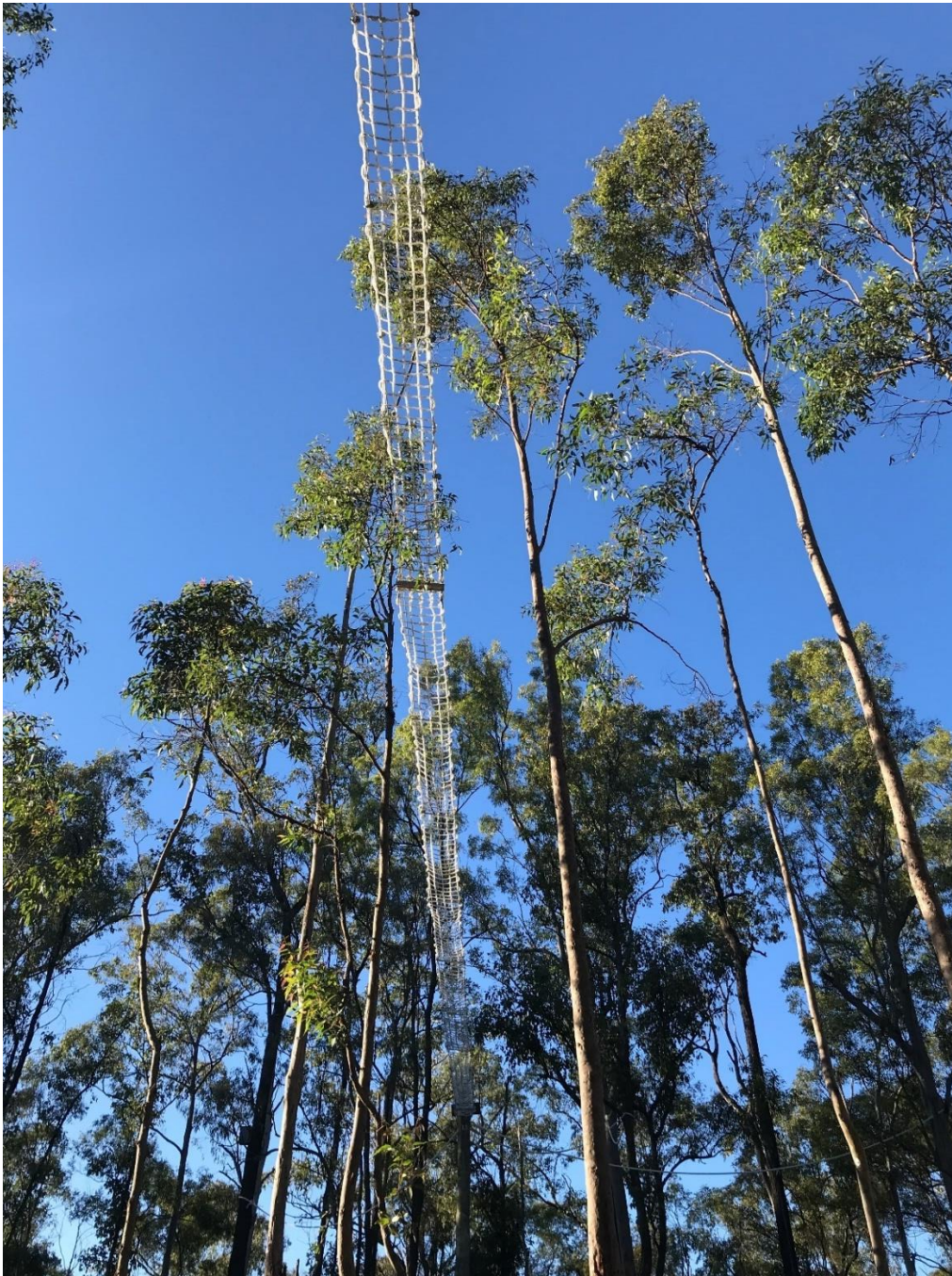
Plate 5.6 Flat rope ladder crossing design Jinker Track, Morton Bay Regional Council (EMM, 2020)
