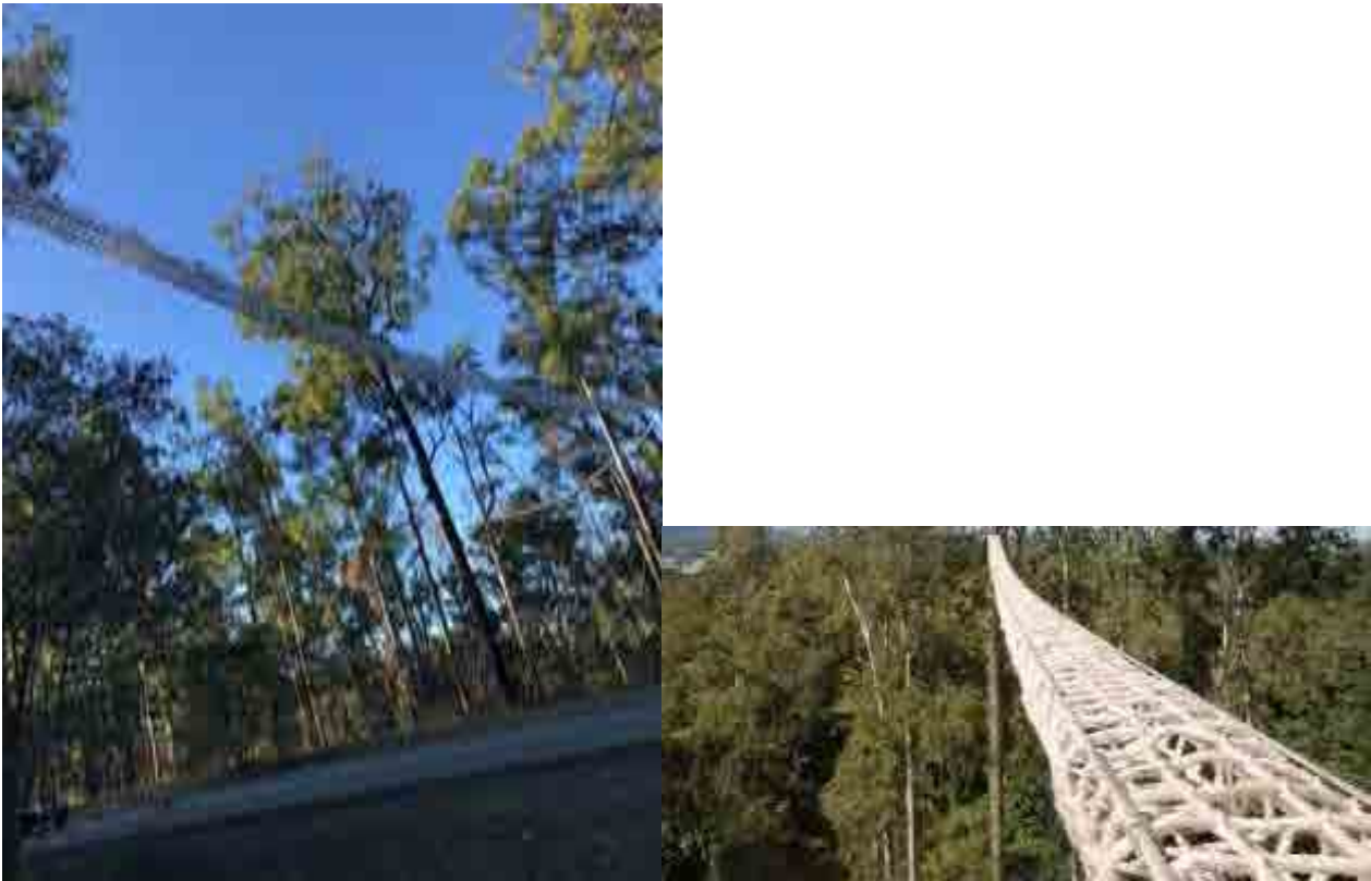
Plate 5.6 Box Rope ladder crossings (image left with cables to adjacent trees) (Left Photo: EMM 2020, Right photo: Fauna Crossings 2020)
